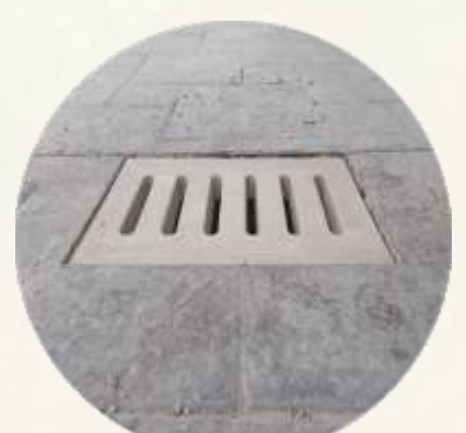
UNDER GROUND DRAINAGE & SEWER
